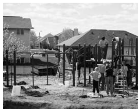
Parents assemble playground equipment at Weber Elementary.
